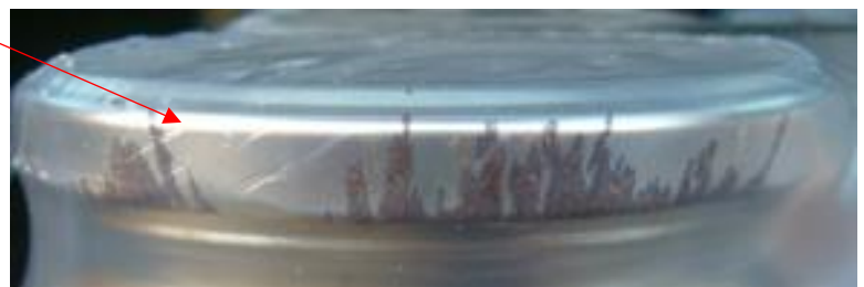
Figure 3: Filiform corrosion example
